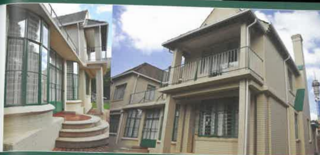
10 Park Lane, dates from 1902 but successive additions record the architectural styles over its lifetime.
